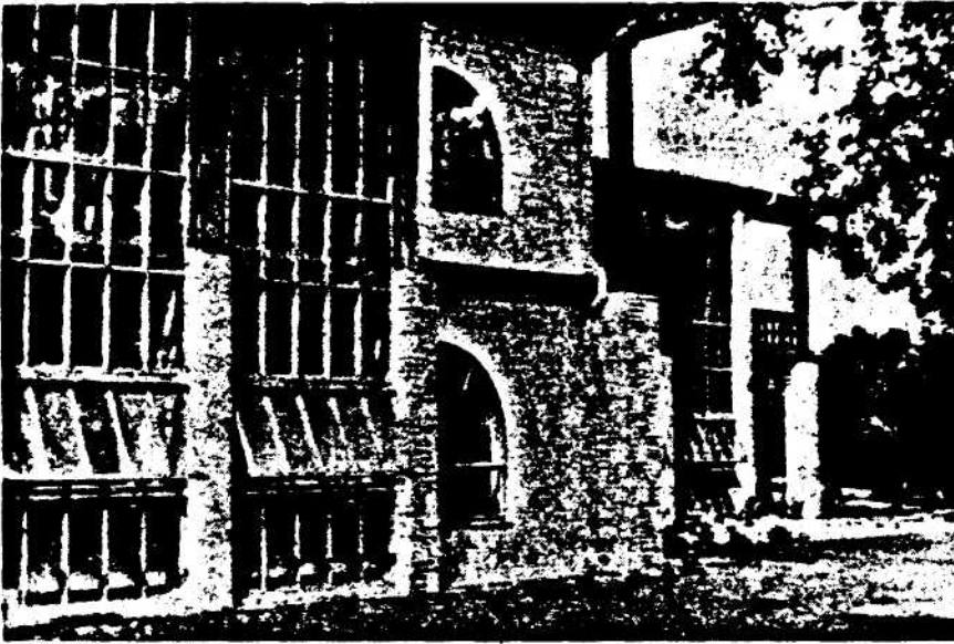
Home for abused and neglected children built from caliche block. Designed and engineered by CMPBS.
