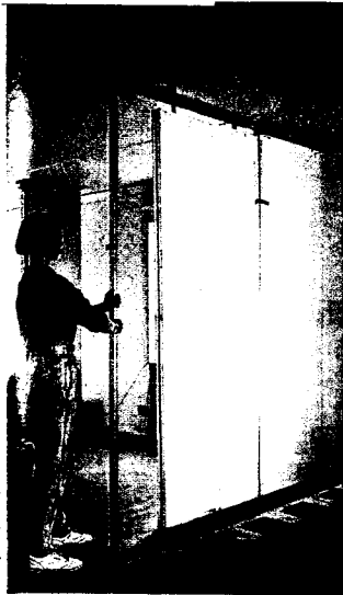
Movable walls held by spring-loaded supports, snap-on wiring channels, and clever plumbing runs add up to
