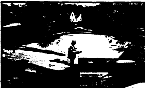
BEFORE: Ponded water on roof decks leads to membrane and insulation deterioration and subsequent leaks.
